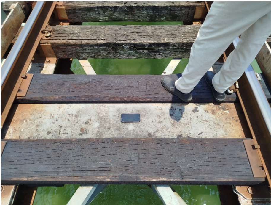
Figure 8: Smartphone fixed on the Cross girder (Source: [8])
