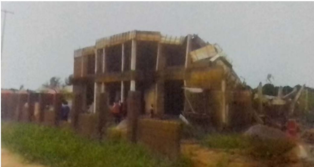
Plate 2: A scene of the Collapse Building Structure (Job, et al, 2019)
