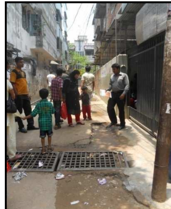
Photo 4: Poor road Surface
