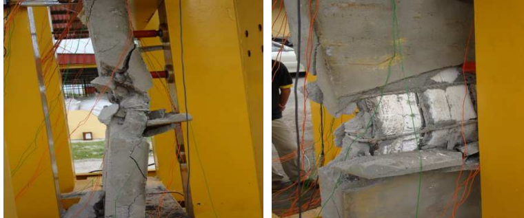
Figure 6: Crushing at mid-height of panel PA-9 due to buckling in the middle zone of panel
