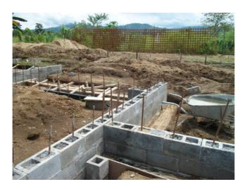
Figure 1: Seismic Designed Cement Hollow Block Wall
