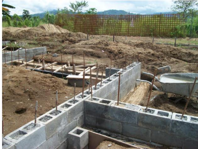
**Figure 1:** Seismic Designed Cement Hollow Block Wall
