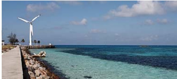
(b) Pulau Layang- Layang, Sabah, Malaysia Average Annual wind speed > 4 m/s
