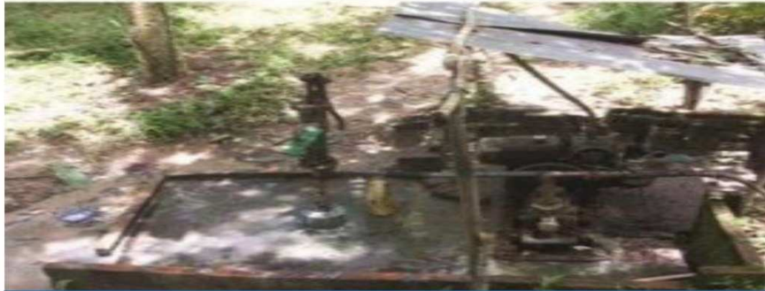
Figure 7: Setting Water Pump for daily drinking water and other activities for the Indigenous Community inside the Lawachara National Park.
