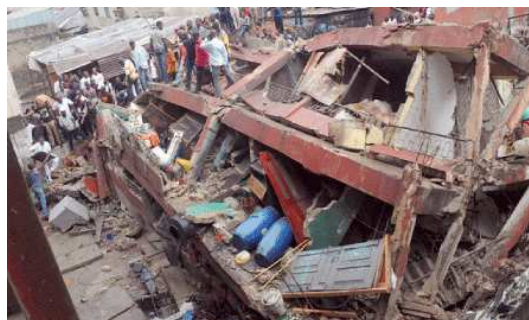
Plate 1: Rubbles of Collapsed Building in Lagos Source: [5]
