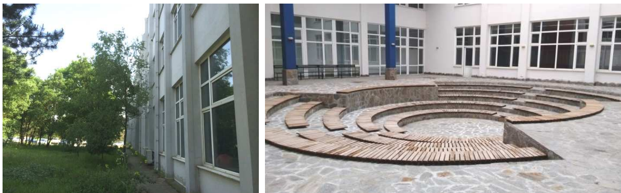
Figure 8: SE Facade of Industrial Engineering Faculty and Open Courtyard
