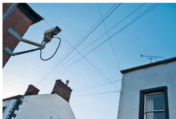
Figure 9: Preventive action: video surveillance cameras enhance public safety
