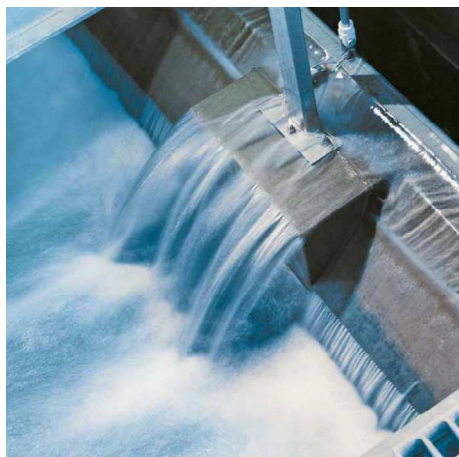
Figure 12: Effective water management: An essential issue for city infrastructures
