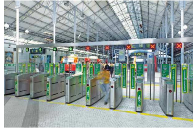
Figure 4: Lisbon: eTicketing and smart systems support intermodal travel
