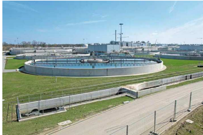
Figure 13: Clean water for Warsaw, Poland: Czajka Europe's largest and most modern wastewater treatment plant.
