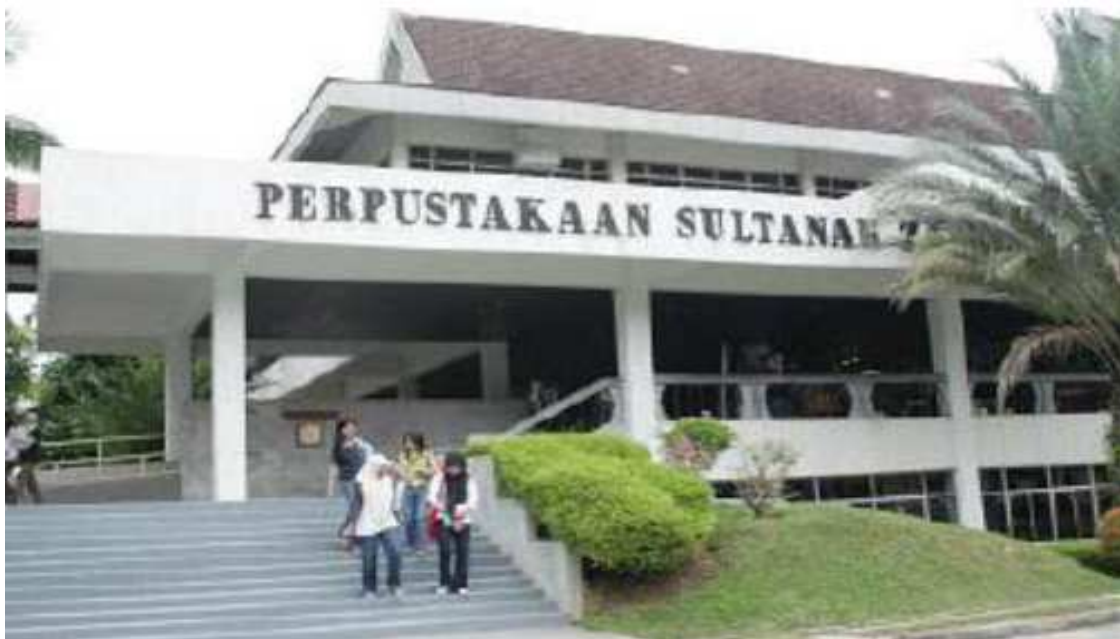
Fig 2: Exterior view, PSZ library (Field Survey, 2012)
