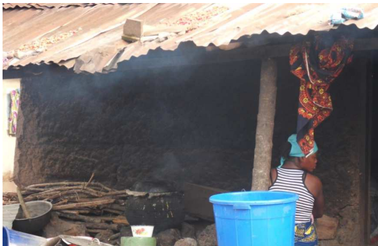
Figure 2: A cooking space attached to the external building wall
