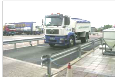
Figure 8: Instrumented Road Pavement Test Site – Aggregate Industries UK [6].
