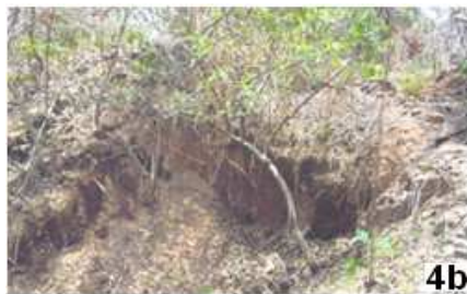
Figure 4b: Pit overburden sliding and rock fall.
