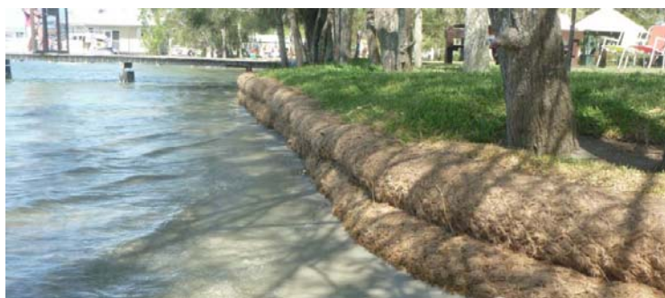
Figure 2b. bank stabilisation using coir logs, Australia (aussieenvironmental.com.au)
