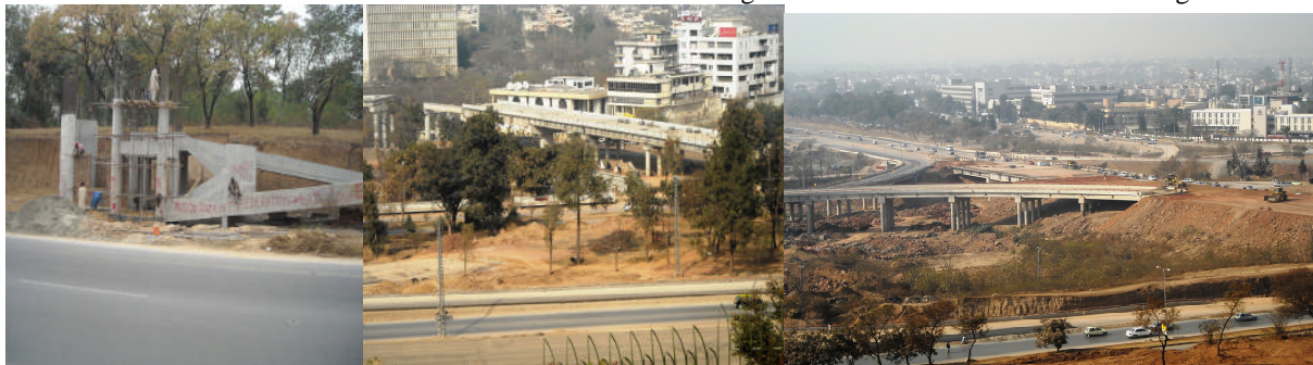
d. Unnecessary use of concrete in pedestrian crossing. e. Visual quality of many building damaged
