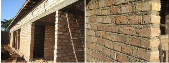
Figure 10. Excessive use of mortar due to uneven sizes/shapes of bricks. Source: The authors.
