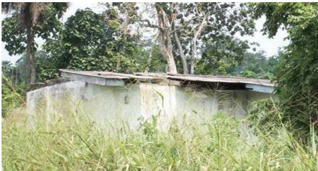
Dilapidated building at the grave site of Bilikisu Sungbo (Queen of Sheba)
